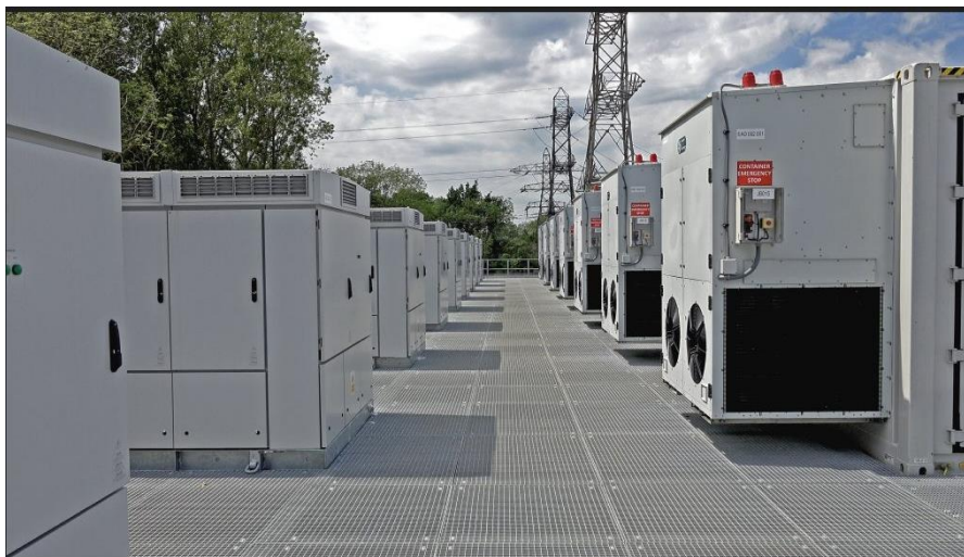
Figure 3-3 Typical BESS configuration
