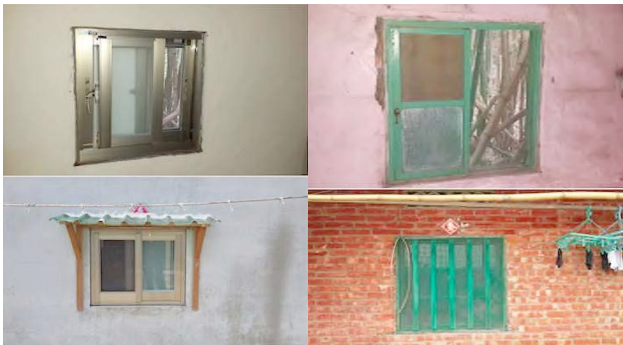
Figure F-1 The picture of the installation of the airtight windows in Fongwei Wind Farm in 03/2014
