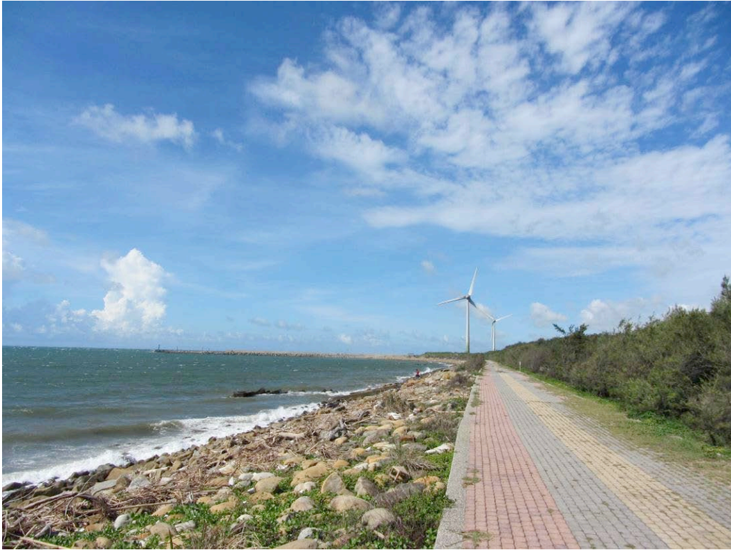
Figure F-7 The landscape picture in InfraVest Fongwei Wind Farm
