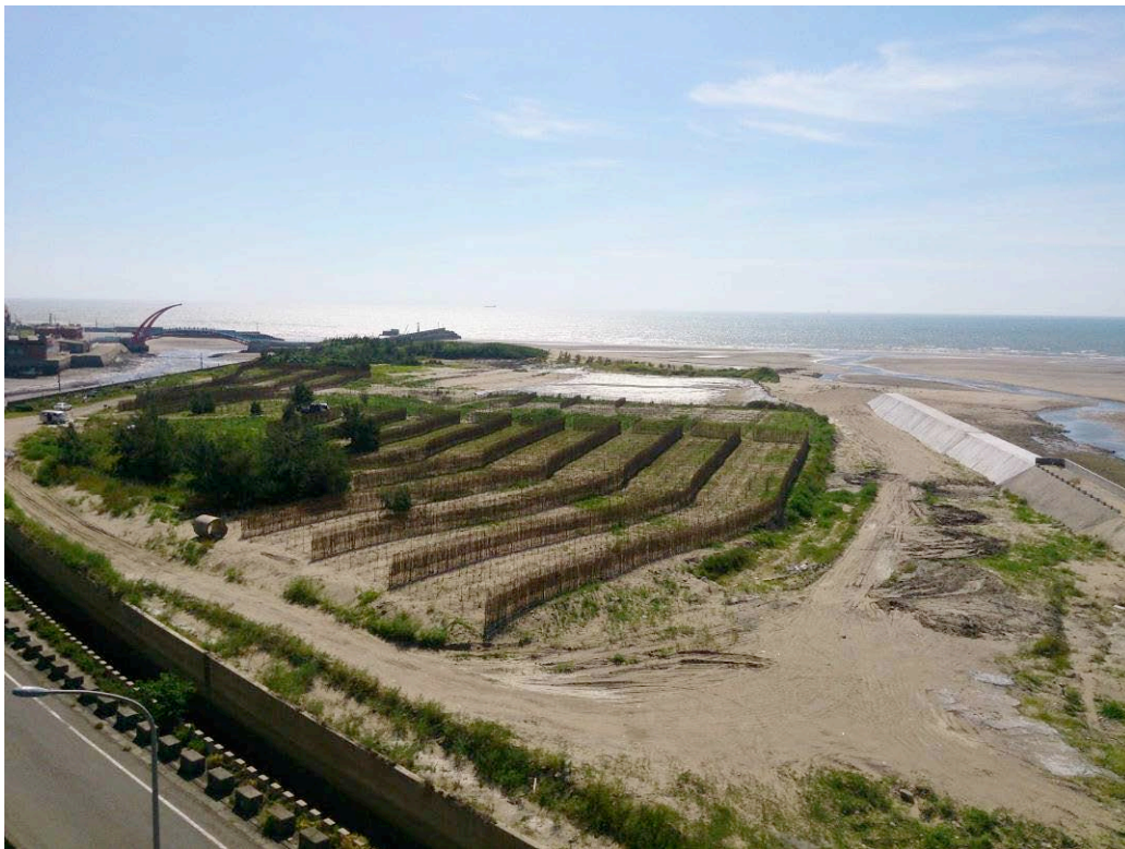
Figure F-3 The re-plantation picture in InfraVest Fongwei Wind Farm
