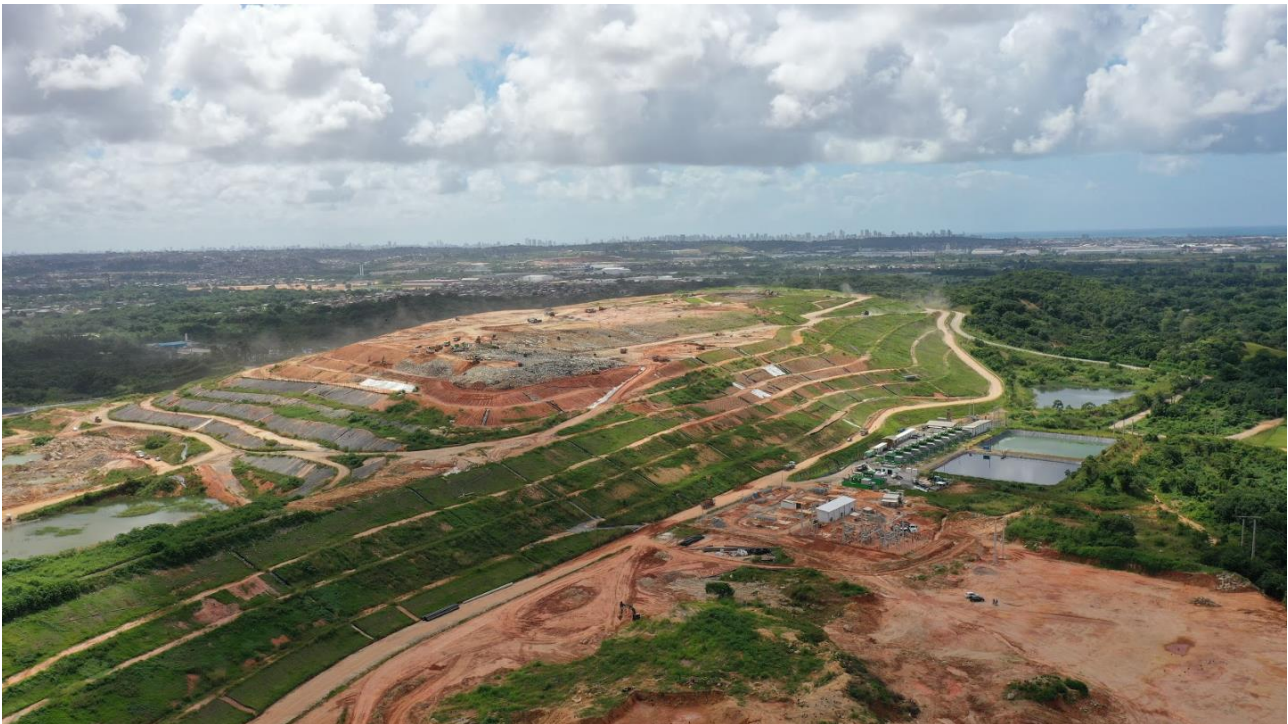
Figure 4 – Panoramic view of the Ecoparque Candeias Landfill Gas Project
