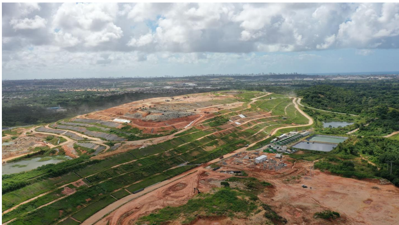
Figure 4 – Panoramic view of the Ecoparque Candeias Landfill Gas Project
