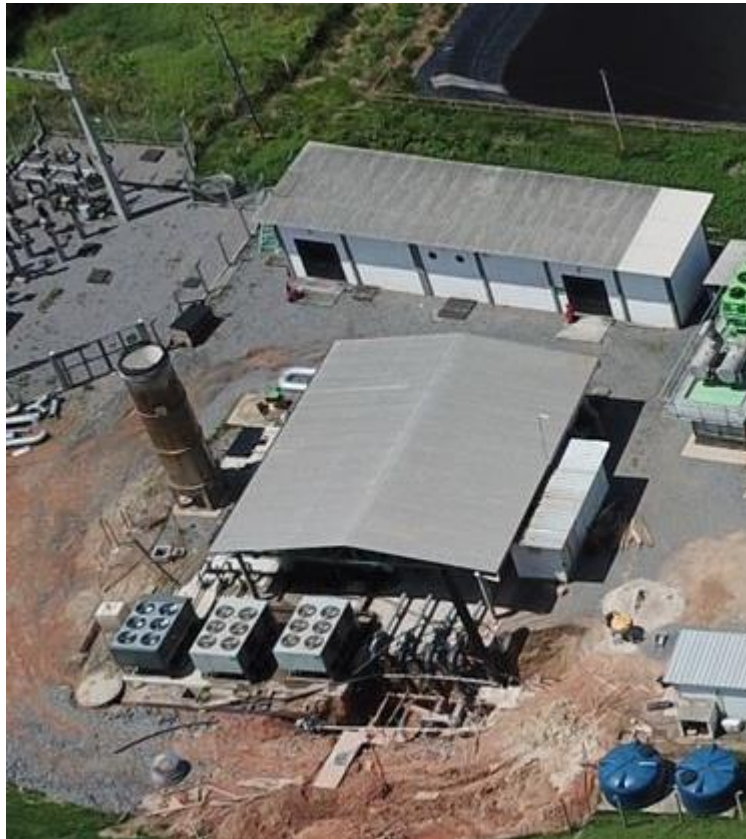
Figure 4 – LFG Flare Station in the project activity
