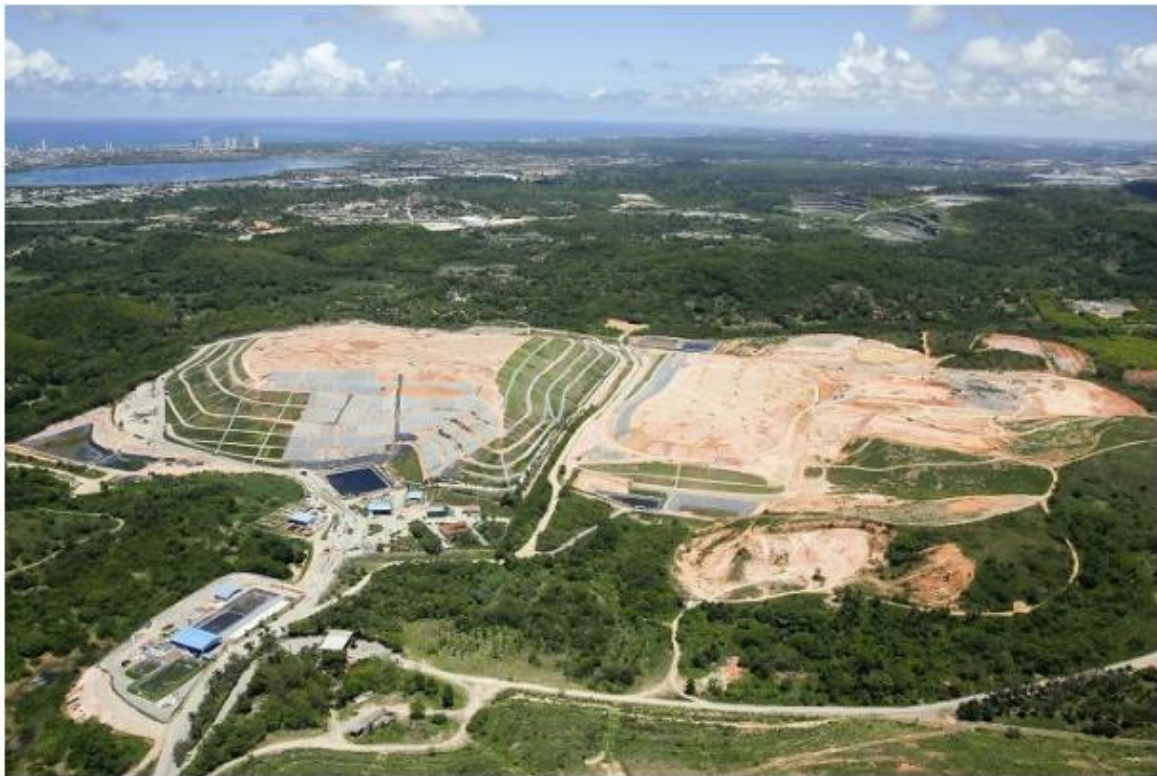
Figure 2 – Panoramic view of the Ecoparque Candeias Landfill Gas Project
