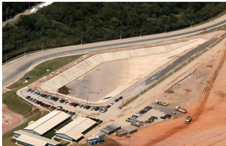
Figure 5 – Leachate drainage system
