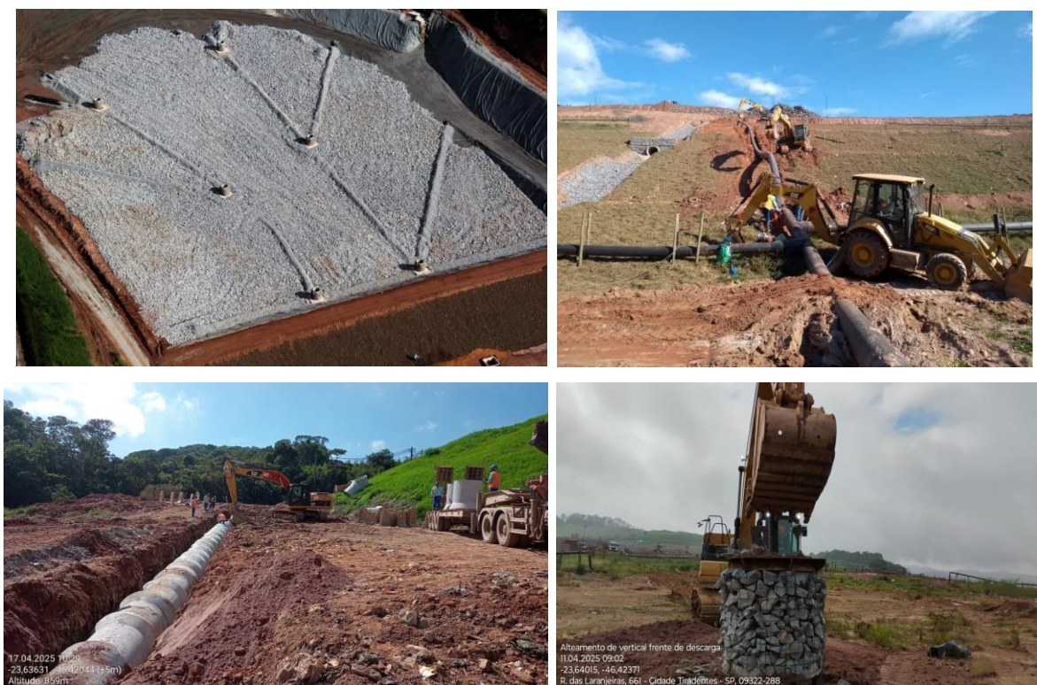
Figure 4 - LFG Drainage System
