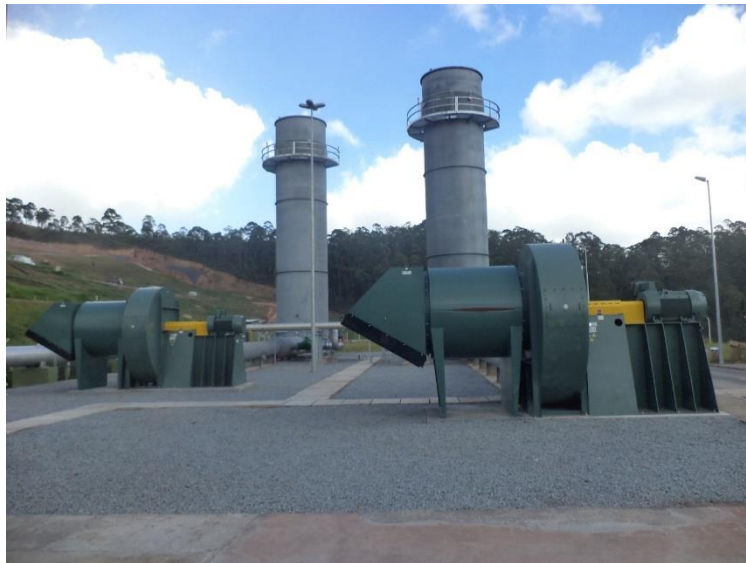
Figure 10 - Enclosed Flare system at CTL Landfill Gas Project (Source: EcoUrbis Ambiental S.A.)
