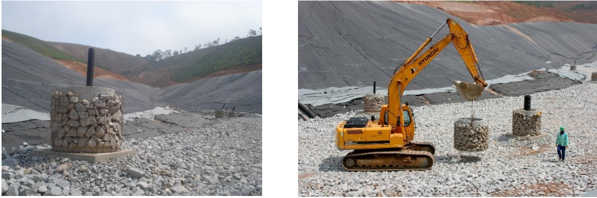
Figure 6 – Design of vertical wells/drains. (Source: EcoUrbis Ambiental S.A.)
