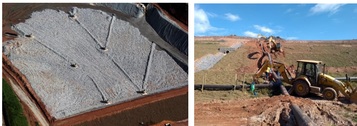
Figure 4 - LFG Drainage System. (Source: EcoUrbis Ambiental S.A.)
