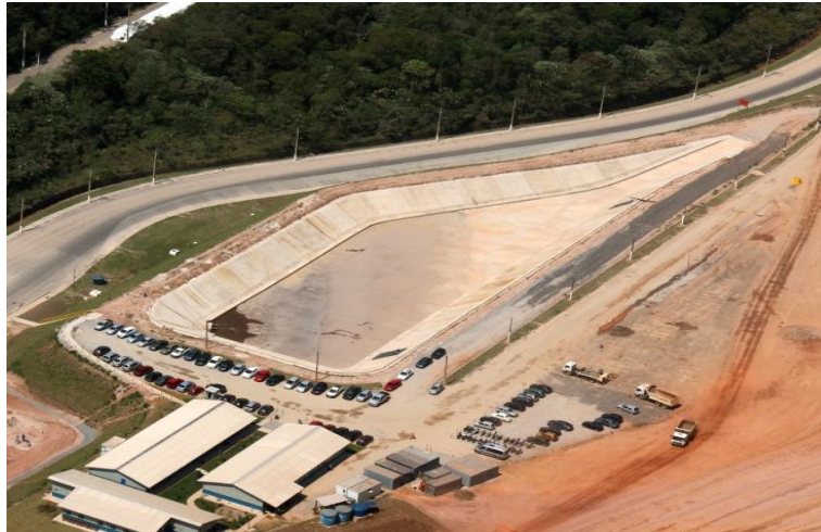
Figure 5 – Leachate drainage system (Source: EcoUrbis Ambiental S.A.)
