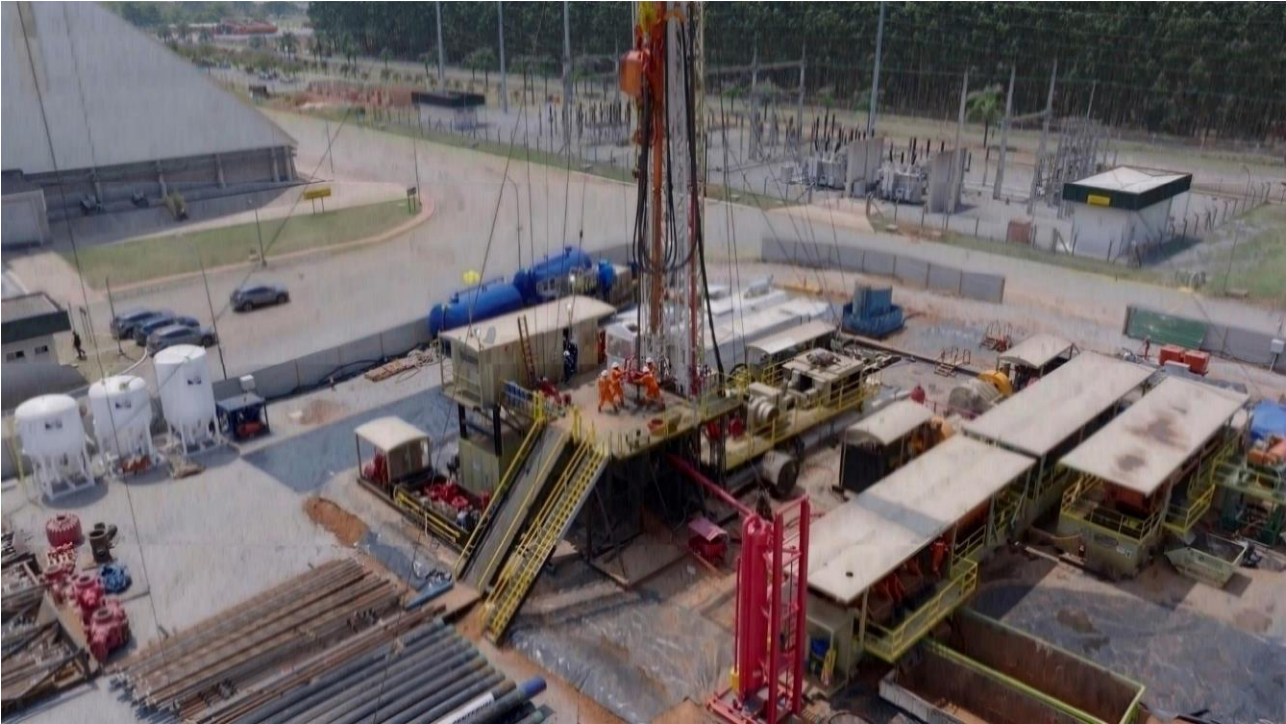
Figure 4. Stratigraphic well drilling.
