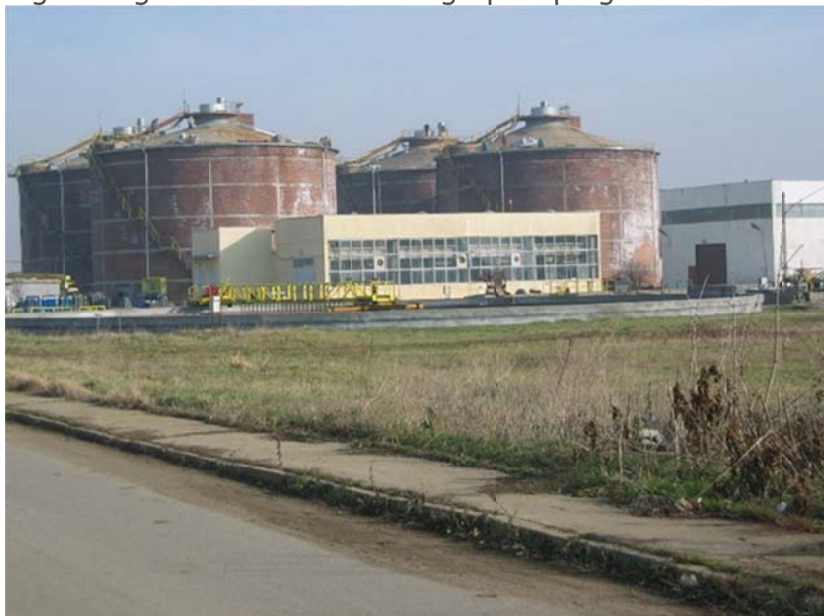
Fig.3: Digesters and raw sludge pumping house
