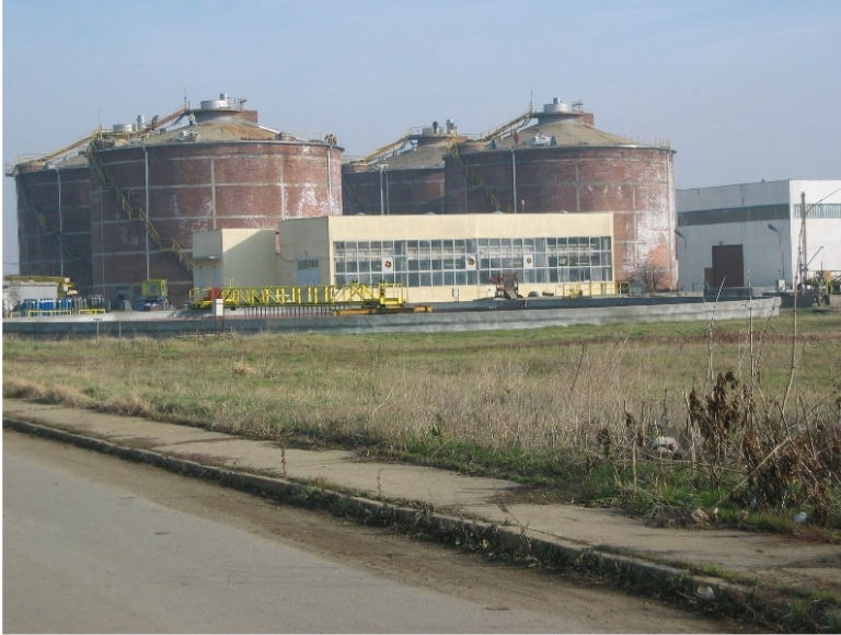
Fig.4: Digesters and raw sludge pumping house
