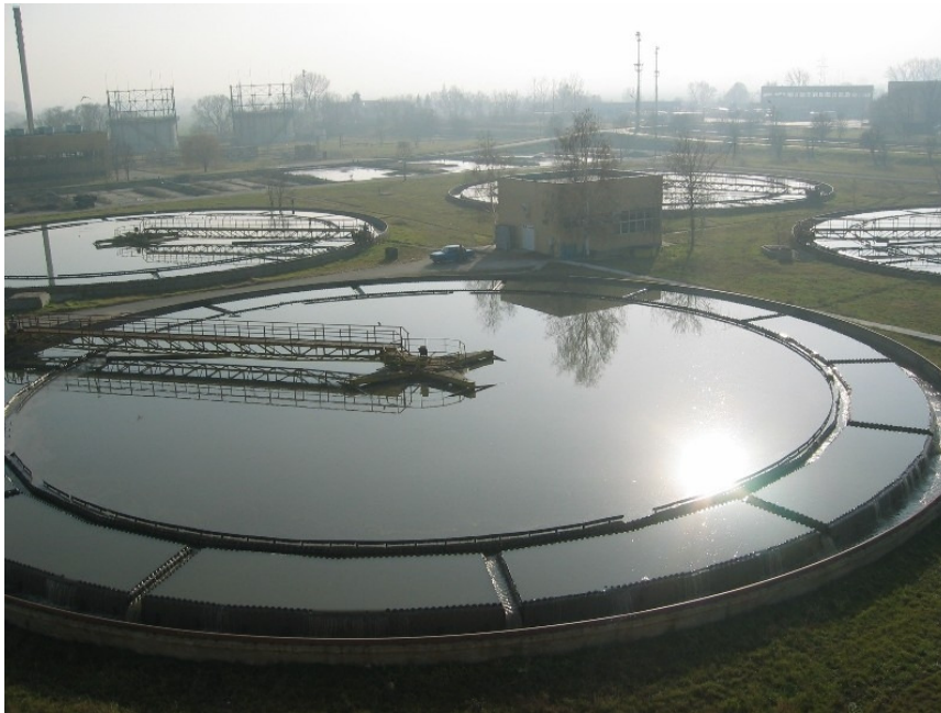
Fig.3: Primary settling tanks
