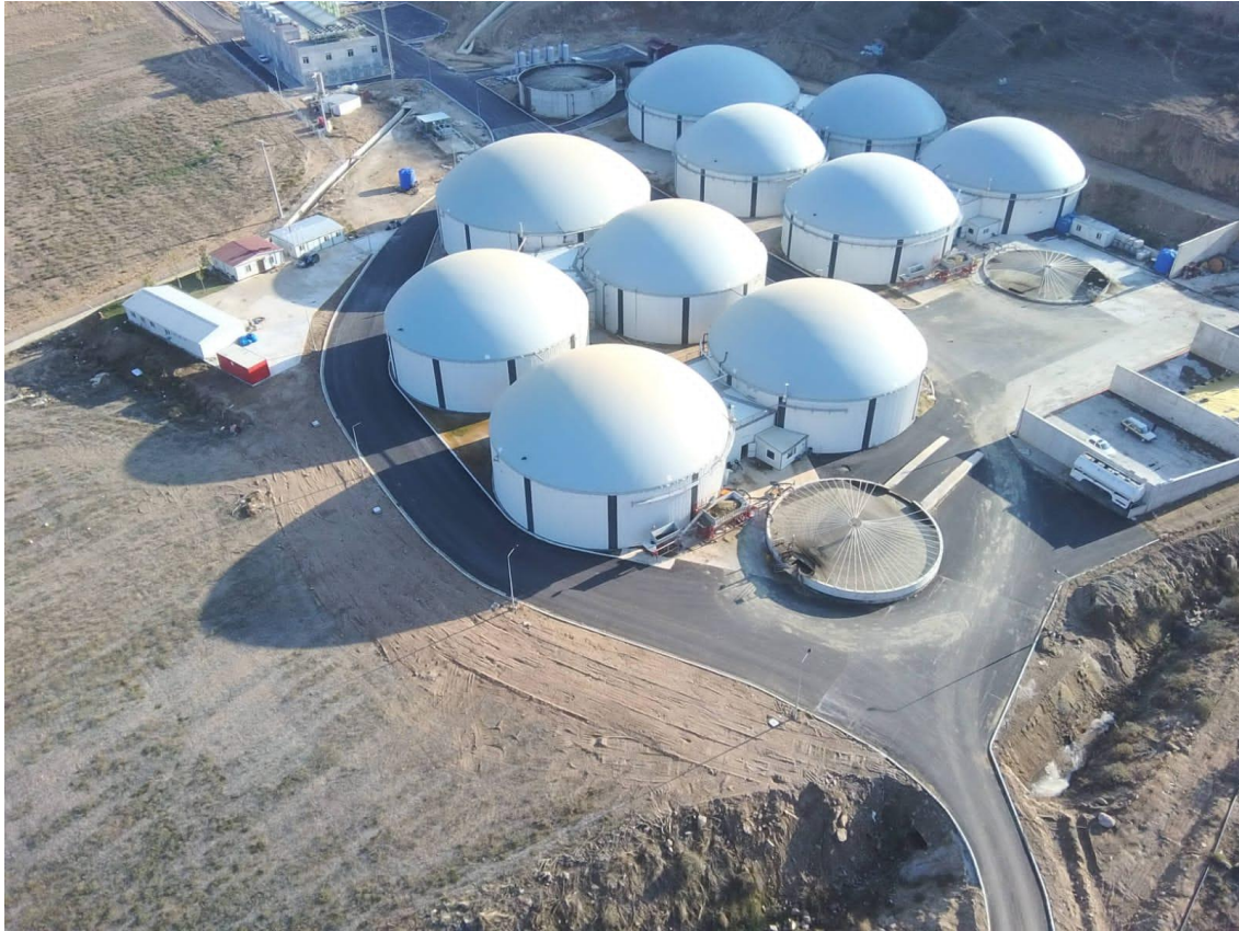
Figure 3. ARF Project Site
