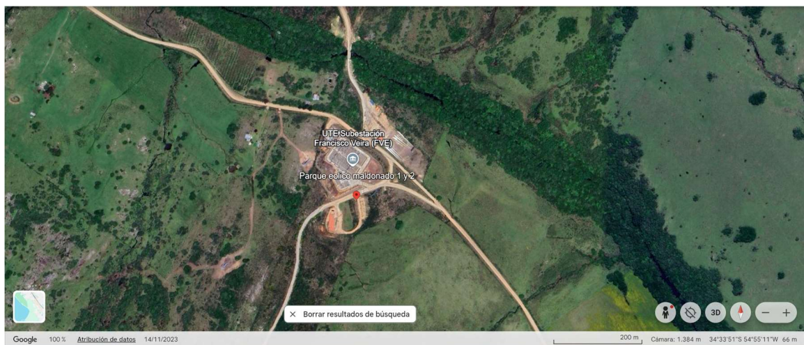
Figure 4 Satellite image of the substation Francisco Veira
