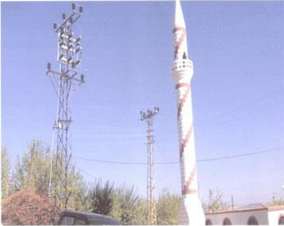
Figure 11 Construction of Minaret of the Balka Village Mosque
