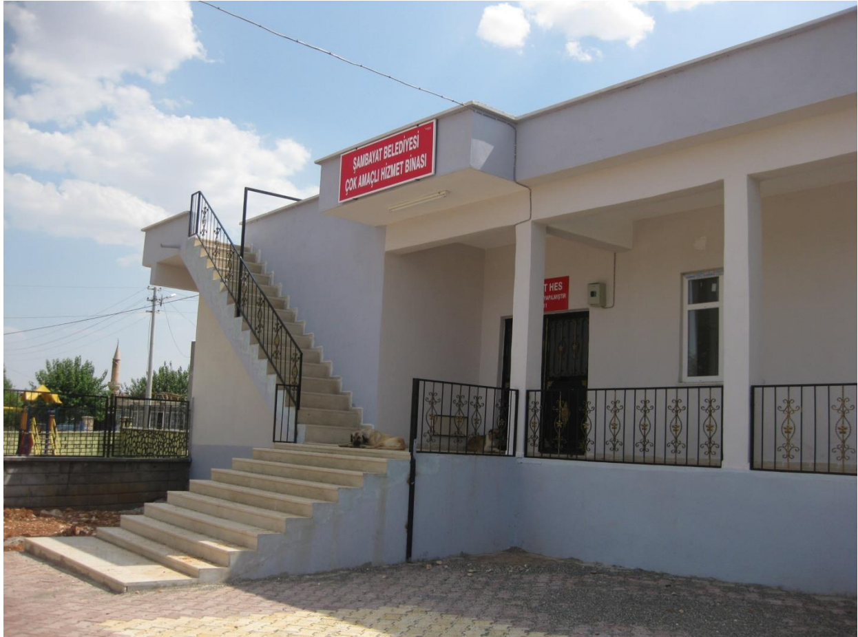
Figure 10 Multipurpose service building for the Şambayat Municipality
