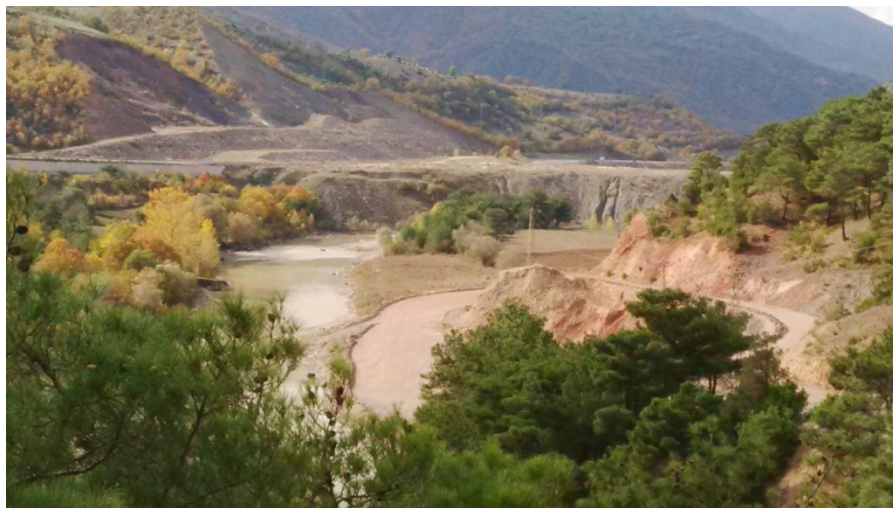
Figure 1: Future weir location viewed from the nearby surface road, image tag: 40°23'50"N 37°19'3"E
