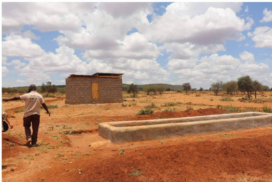
Figure 22. Watering point for animals and building for water tanks for the community
