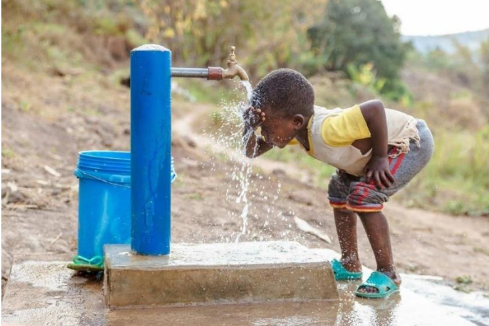
Safe Drinking Water Provision
