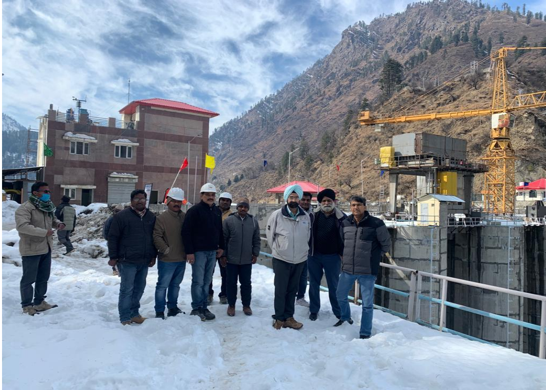
VIEW OF DAM FROM INTAKE SIDE
