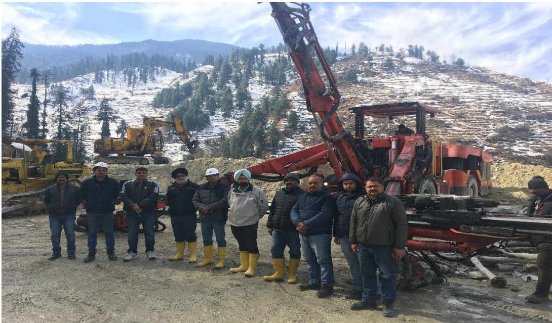
DRILL JUMBO- OUTSIDE ADIT 1 (FOR FACE-3 EXCAVATION BY DBM)
