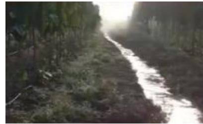
Drainages to control water excess
