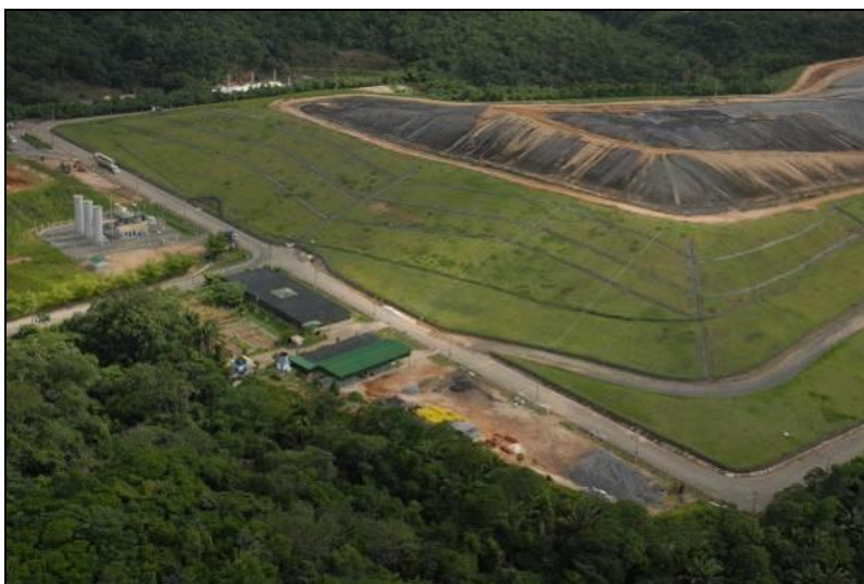
Figure 2: Partial view of the landfill area showing MSW disposal cell (where the project's LFG collecting wells are installed) and the project's LFG destruction station 2
