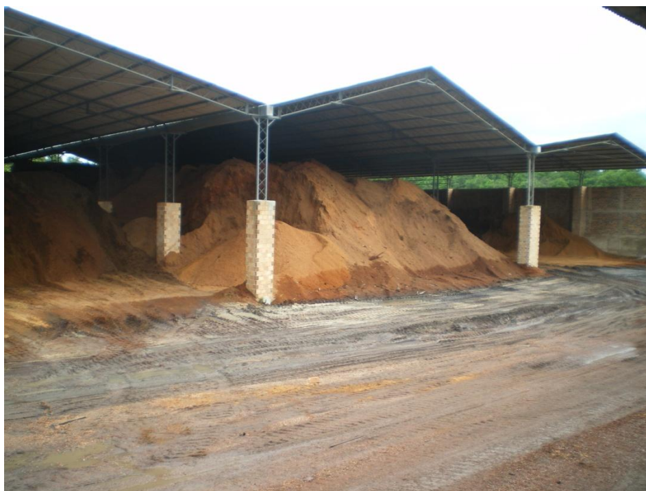
Figure 4: Photo of the shed built. (2011)
