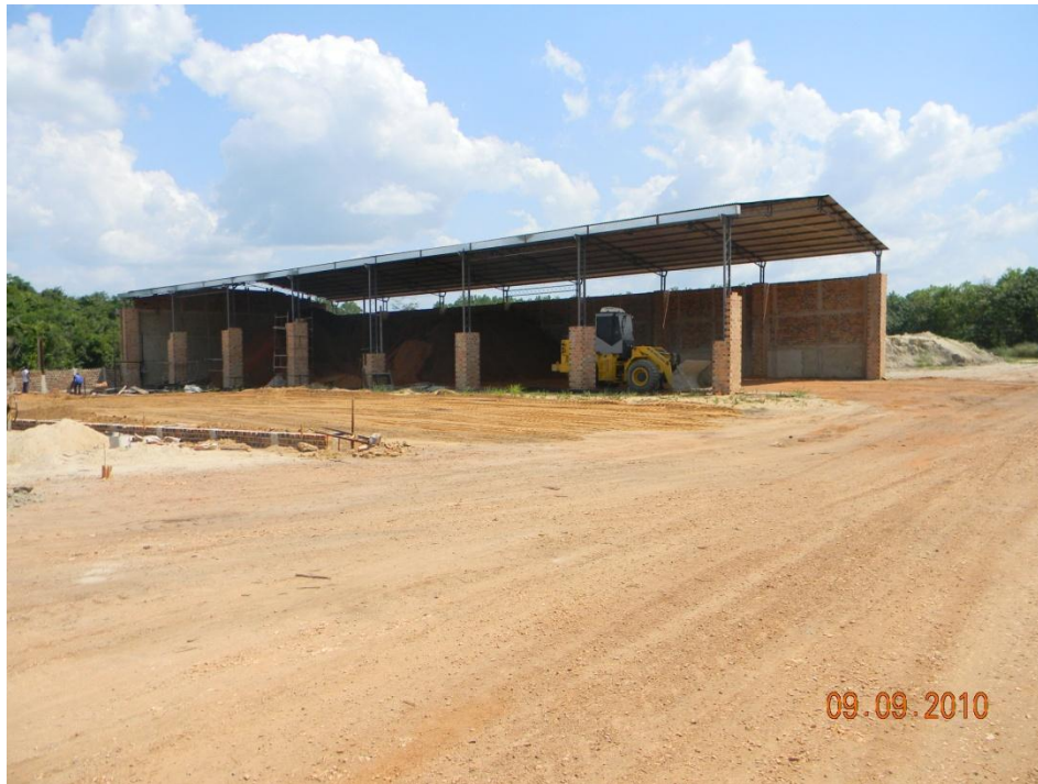
Figure 3: Photo of the construction of the shed.
