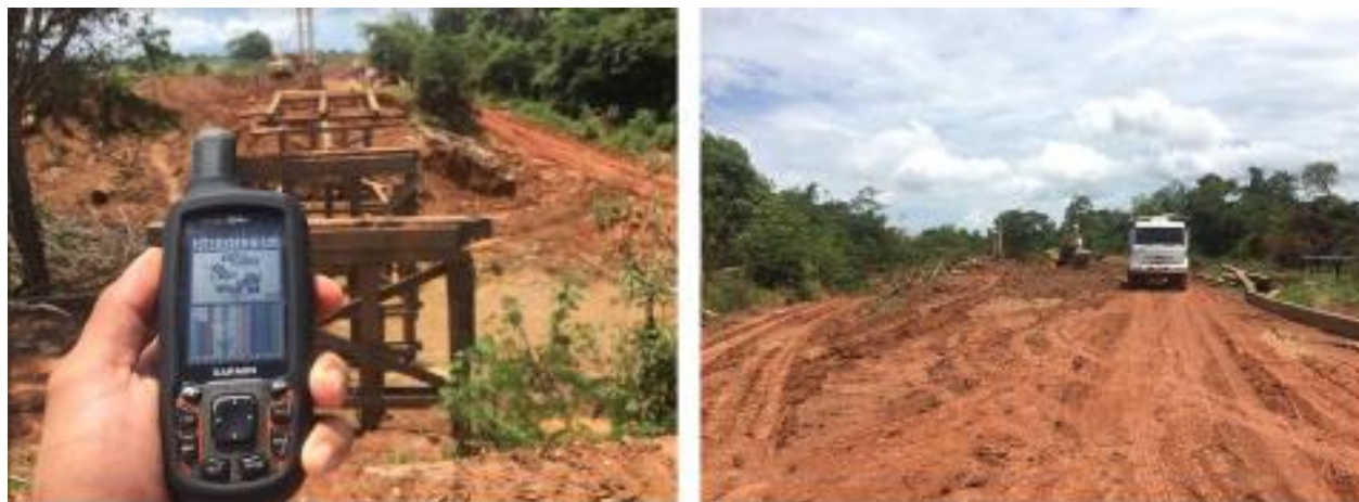
Figure 25 - Construction of the bridge, Mococa Branch Line.
