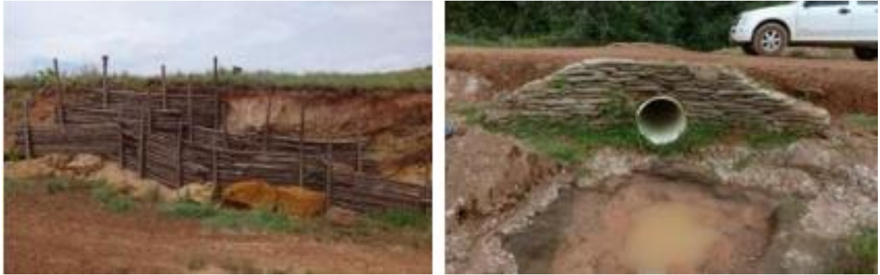
Figure 32. Erosion control program in REFORESTADORA CUMARE SAS
