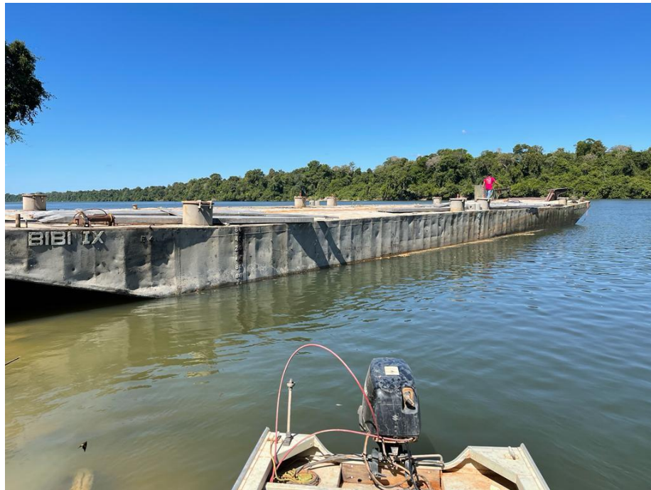
Figure 9. Ferry installed on the Roosevelt River, between Boa Lembrança and São Damião properties
