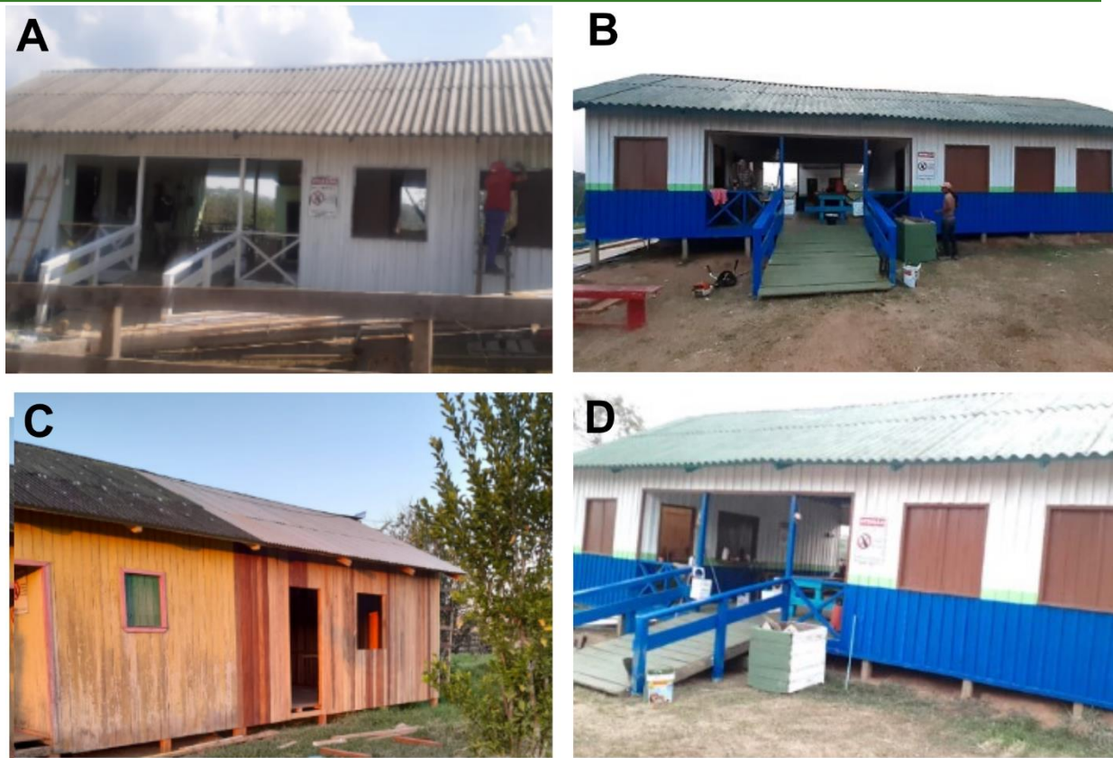
Figure 33. Expansion and renovation of schools in Porongaba.
