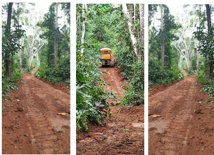
Figure 4 - Maintenance of lanes in Porongaba
