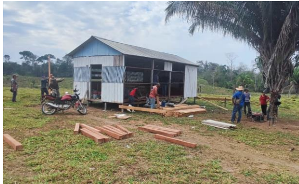
Figure 2 - “Nossa Senhora das Candeias” Chapel renovation
