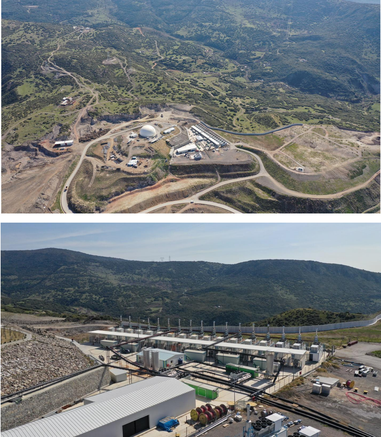
Figure 4. Panoramic of the Izmir LFG project. Source: Google Earth
