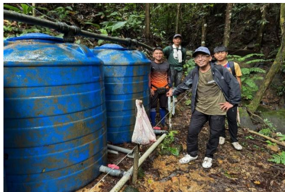
Figure 8: VVB with water tanks in the project
