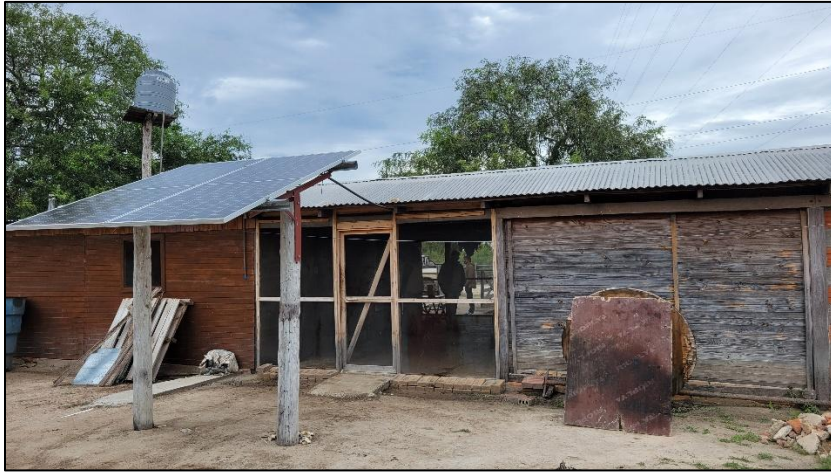
Solar Panels Installed at Guards' House (Photo Credit: Ostrya Conservation)
