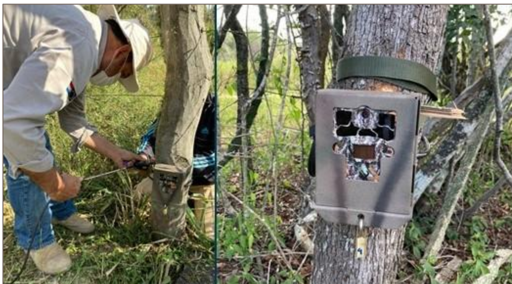
Photo 5.1. Installation of camera by Quadriz staff.
