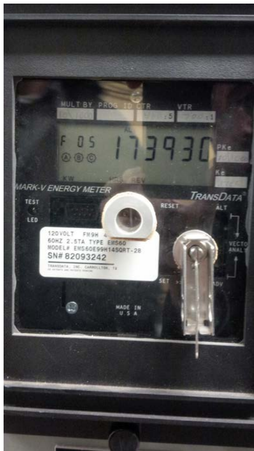
Figure 1 - Custody Meter (SN # 82093242)
