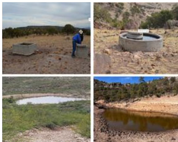
Figure 6: Water Conservation and Storage Structures
