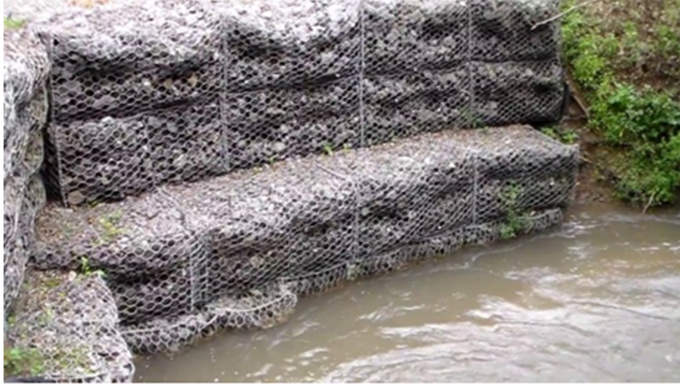
Figure 6: A gabion built on a seasonal stream of a ranch
