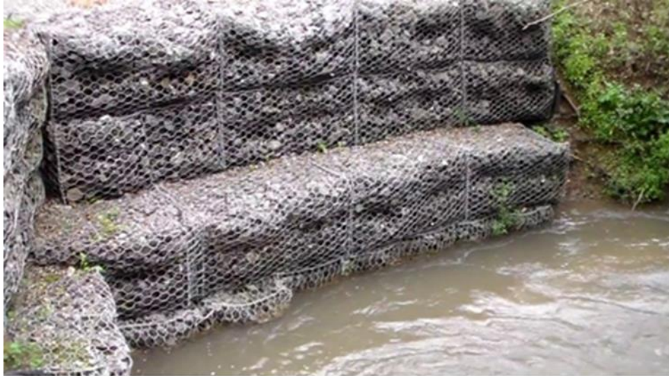
Figure 4: A gabion built on a seasonal stream of a ranch
