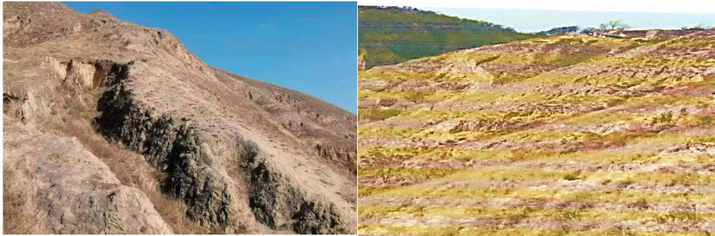
Figure3-2. The degraded land before the proposed project
