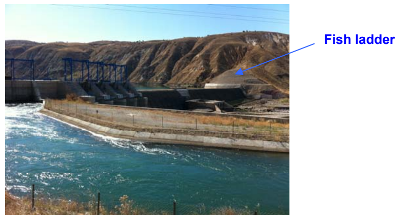
Figure 4. Current work in process of the fish ladder construction. 2
