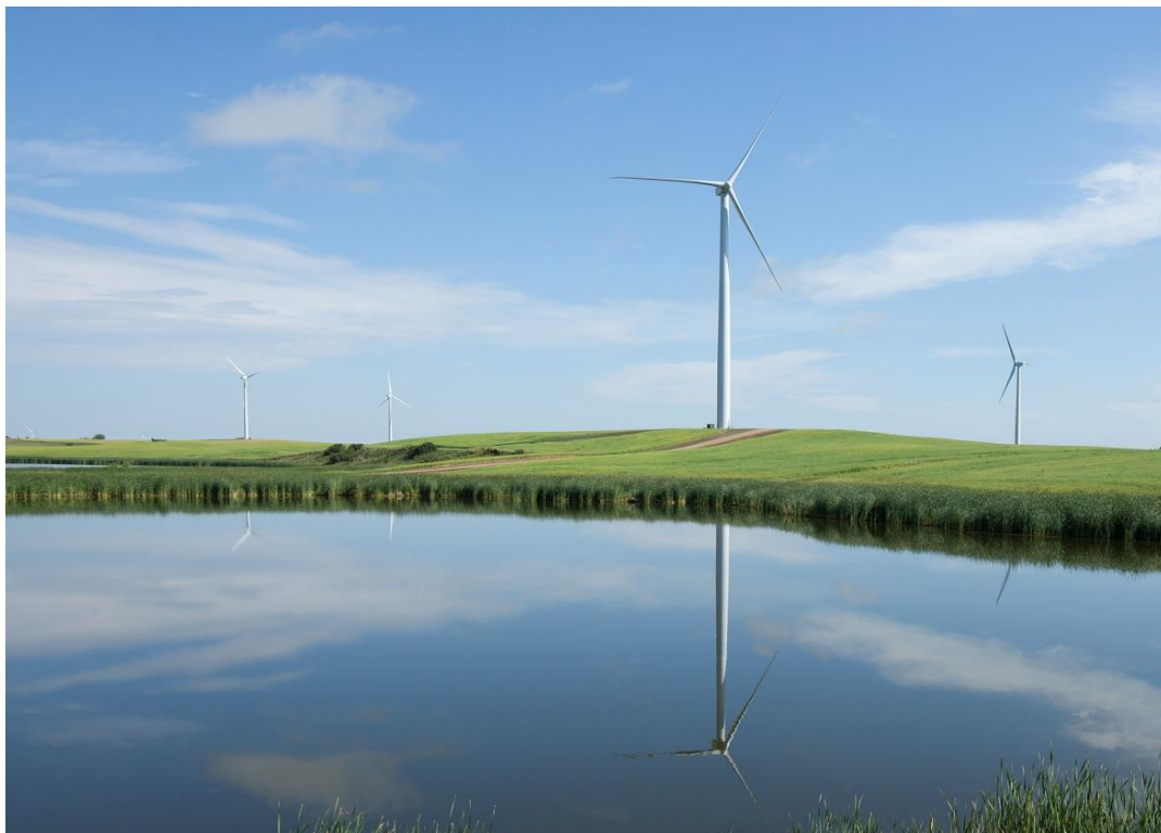
Figure 3 Images of Project
