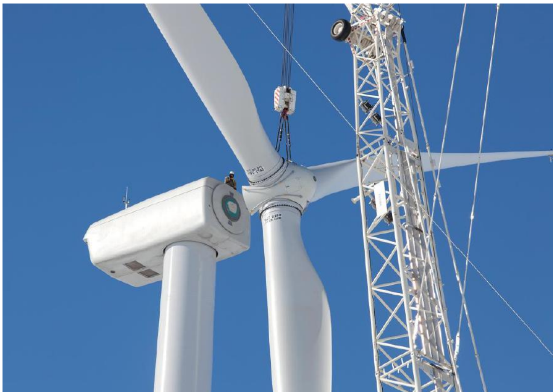
Figure 3 Image of Project
