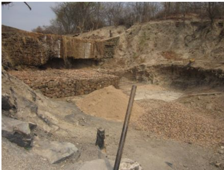
Picture 5: Repairing of the damaged dam wall
