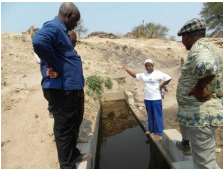
Picture 3: Irrigation restoration
