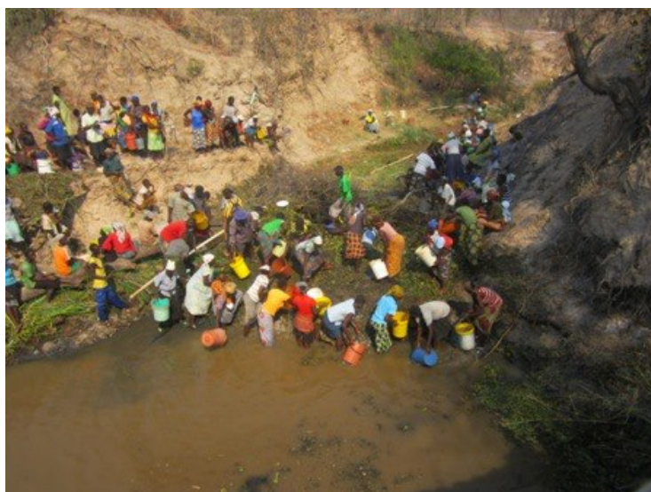
Picture 4: The Community pulling together to drain the eroded area on the other side of the Dam wall at the Tyaba Irrigation Scheme. Set to start doing repairs on wall
