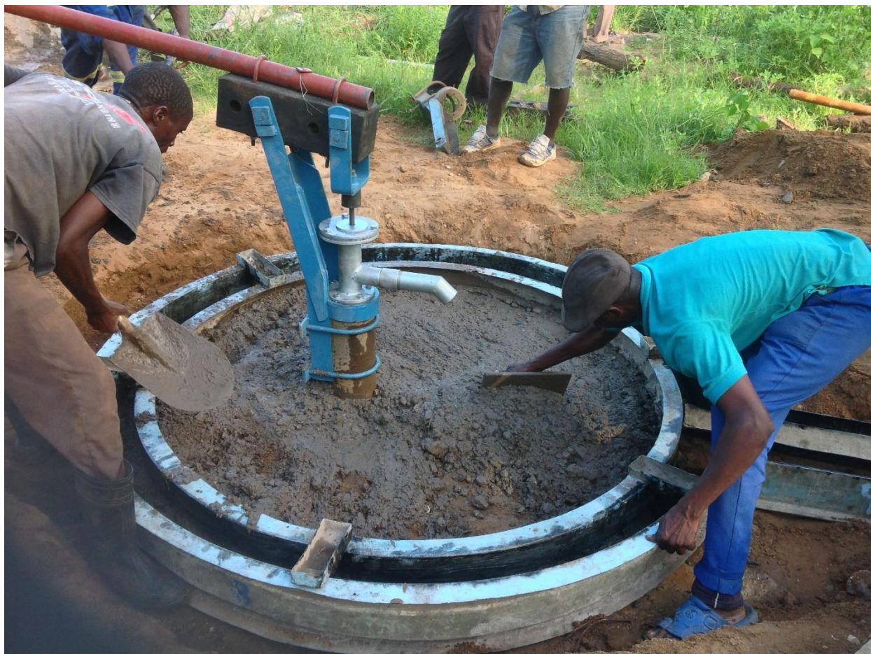
Figure 17: Kariba REDD+ Project borehole resuscitation
