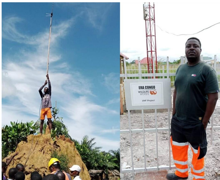
Figure 2.4 The VHF signal being received in Lusaka (left) and the new VHF tower in Inongo (right).
